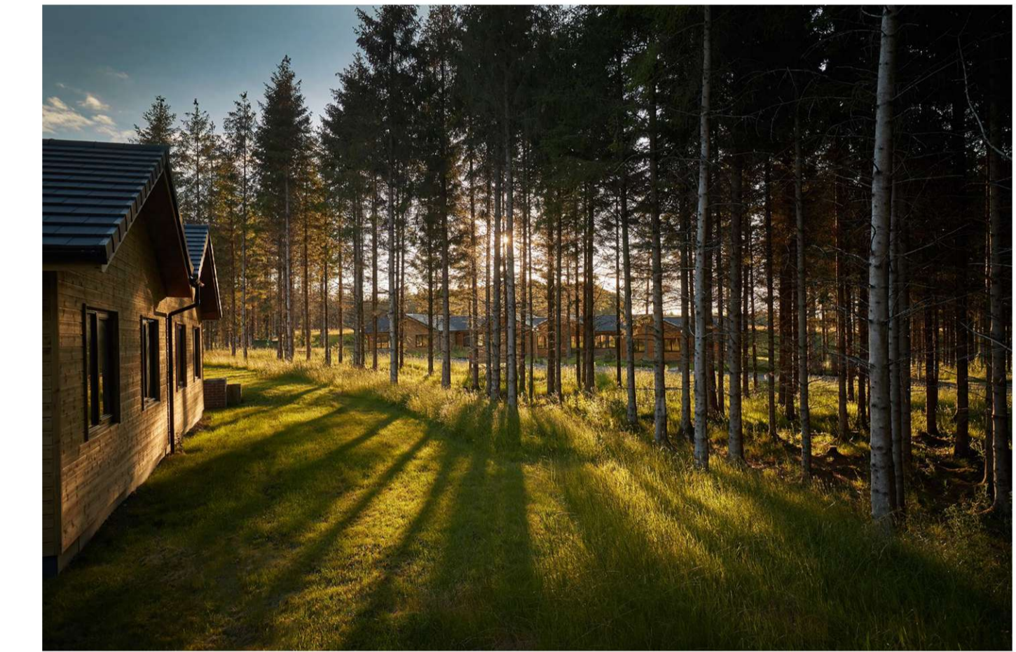
Typical rear of lodge clusters - Longford Forest
